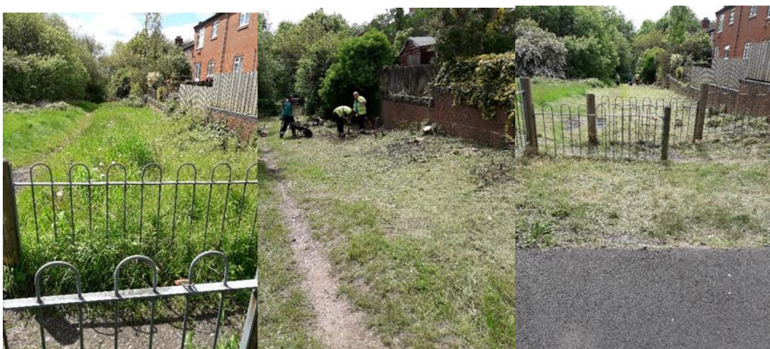
Land to rear of Pearl Mill Close before and after
